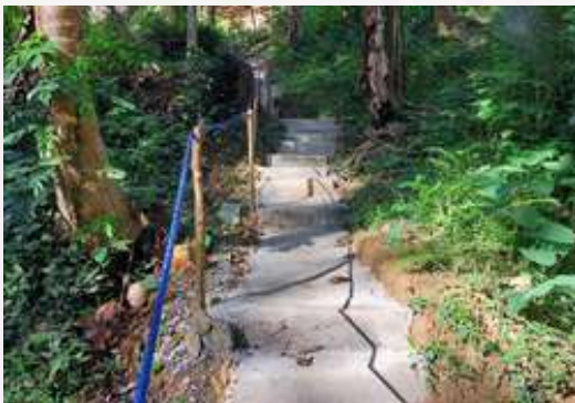
New trail to MBCC. Photo by K. Cielo.
