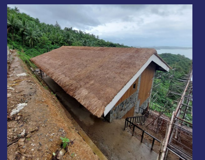
MBCC construction progress
