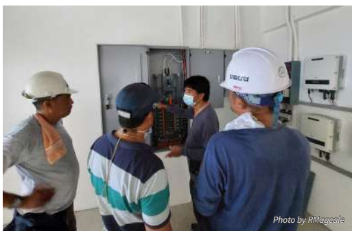
Inspection at the Utility Building
