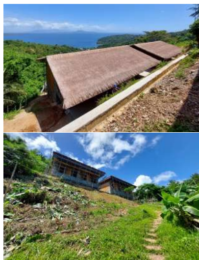
Construction progress of MBCC Phase 1
